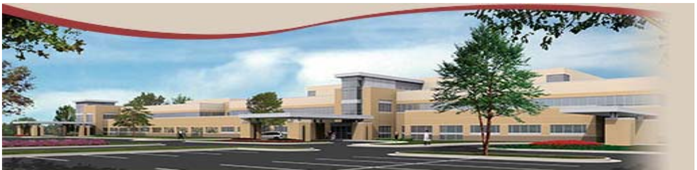
The brand new Southwest Health Center located on Eastside Road within sight of the Platteville Industrial Park.
